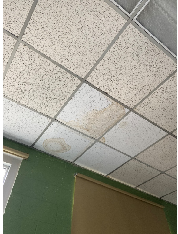
Figure 4 Stained Ceiling Tiles from Water Leak in Classroom
