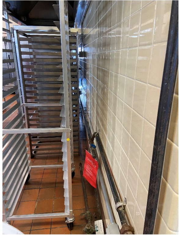
Figure 1 Capped Gas Line in Kitchen
