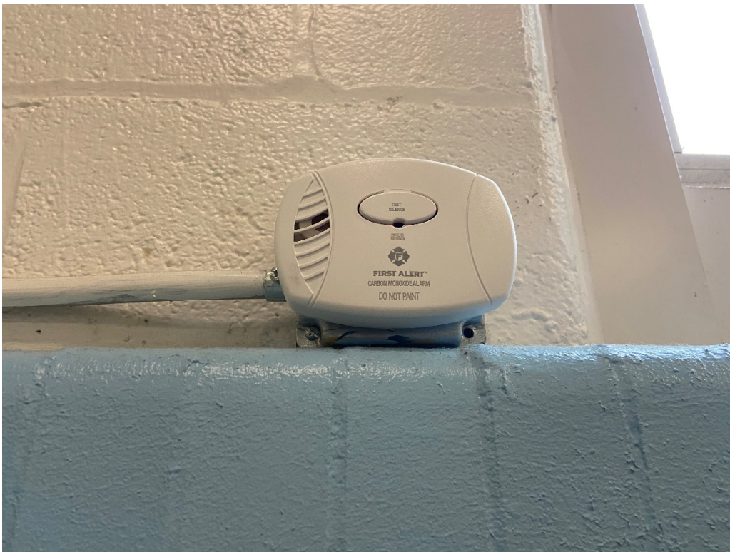
Figure 3 Carbon Monoxide Detector in Cafeteria
